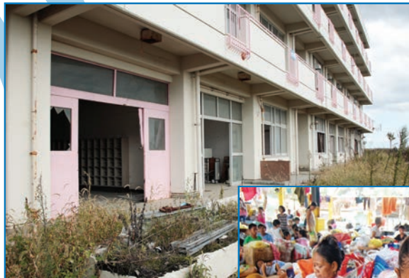
Left: Arahama Elementary School building was damaged by tsunami in Sendai, Japan.
